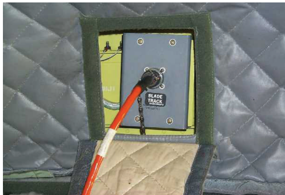
Figure 4. BLADE TRACK Bulkhead Receptacle Near STA 256
